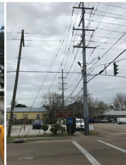
Figure 23. Existing Conditions. Poor drainage, undesignated egress and ingress, missing curbs and
