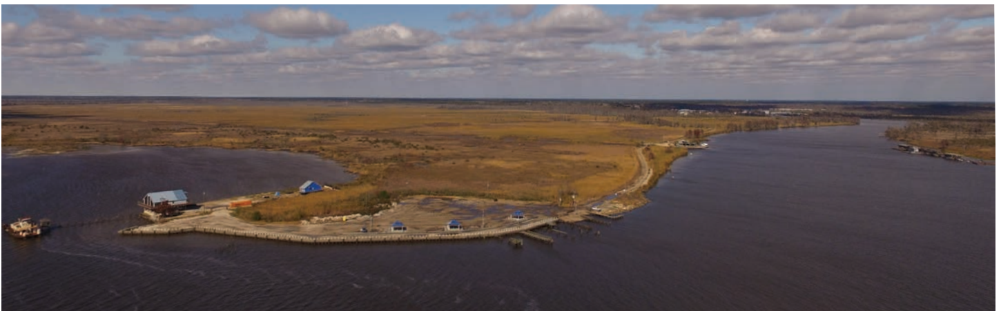
Existing conditions at the lakefront boat launch
